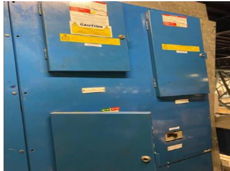
Existing Ottermill switchgear
