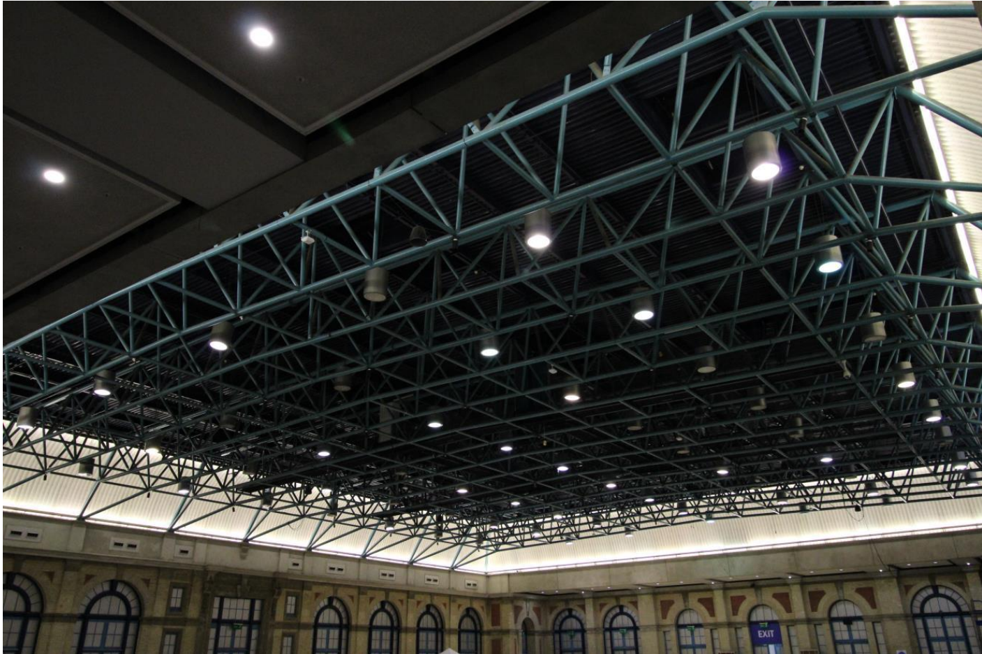
Photograph I – The West Hall is approximately 50mx50mx30m
