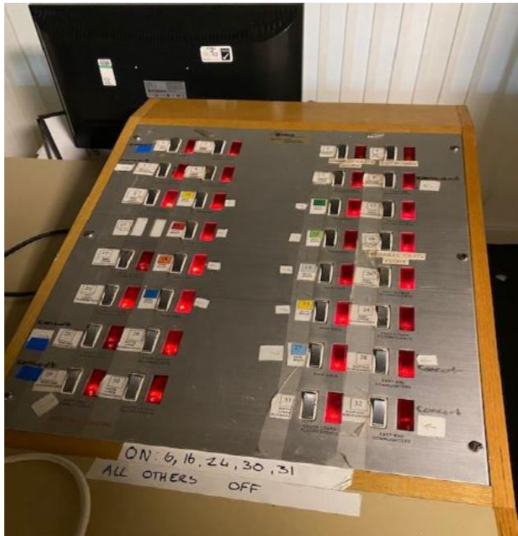
Existing Lighting Control desk
